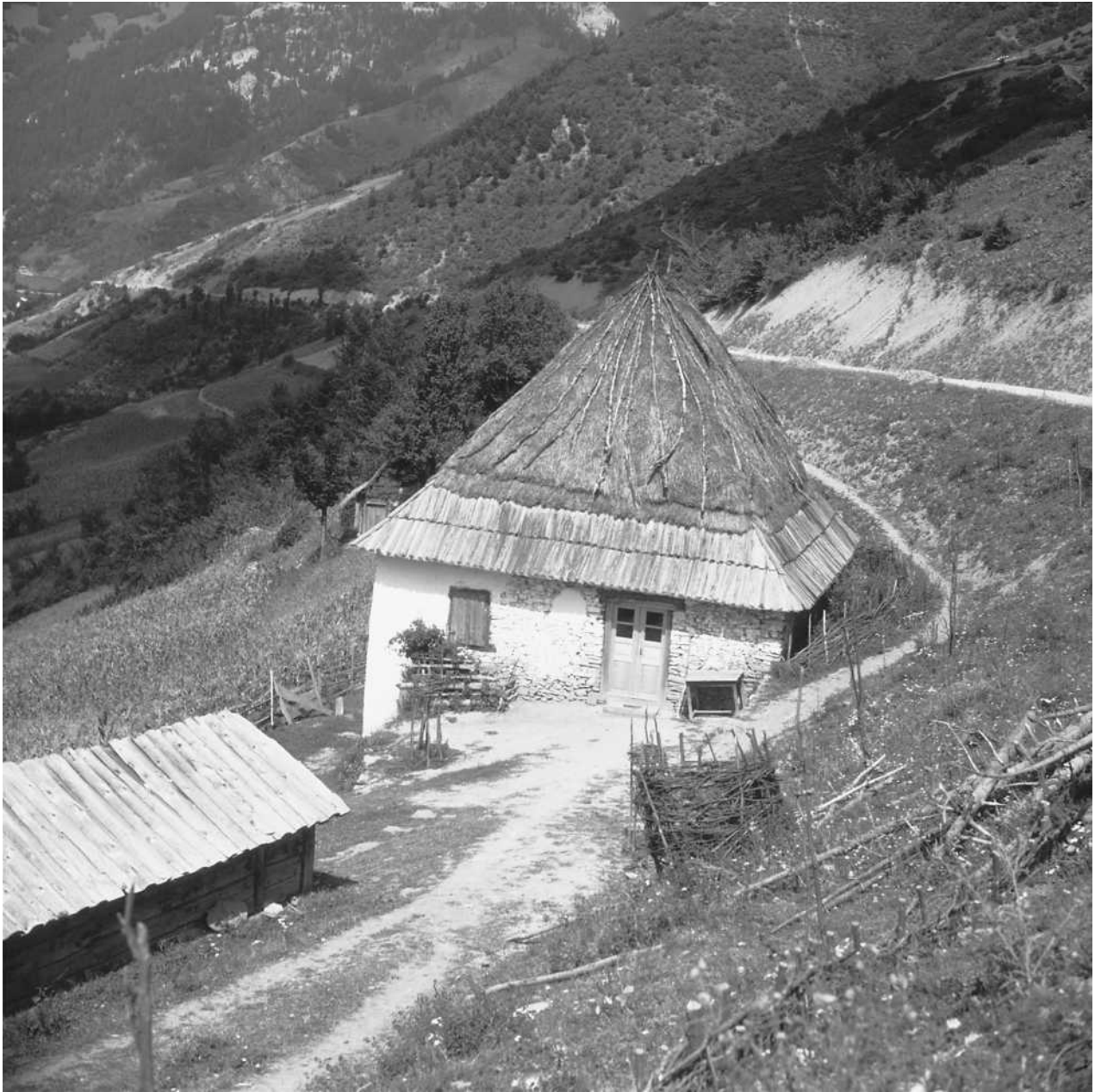
A typical house in Montenegro. Most houses in rural areas are still relatively close together.
